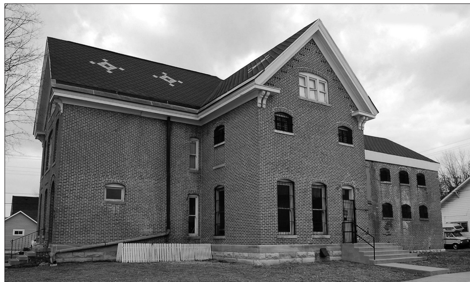
The old Morgan County Jail and Sheriff's Residence — as seen in this 2011 photo — was in need of some repair work but still structurally sound. Its original construction was completed in 1890, and it was used as the county jail for more than 100 years. It has since been refurbished and repurposed, now serving as senior living apartments. But many of the bars on the windows remain in place as homage to its former purpose. (Earl Leatherberry courtesy photo)
